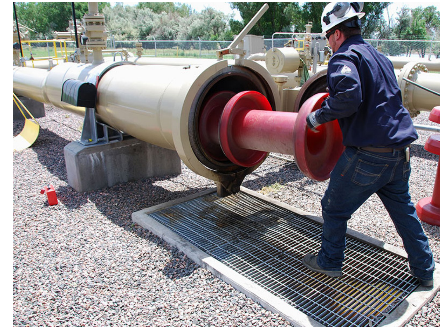
Billy Ops, putting Pig in pipeline
